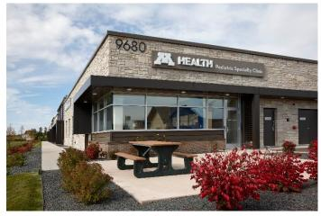
The ACM-2000RS Series is our **most economical** rain-screen panel system, which provides a contemporary look with <u>crisp, caulk free edges</u>. ACM panel systems are best used in low rise applications above grade. The ACM-2000RS system is designed as drained/back ventilated system. This system utilizes integrated aluminum plate attachment flanges for <u>faster installation</u> than spline joint rainscreen systems.
