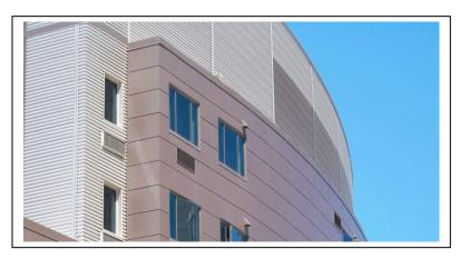
The AP-2500RS Series is formed plate, **back-ventilated rainscreen** panel system, which provides a smooth joint with caulk free edges. AP panel systems are best used applications that go down to grade, or as accents with low volume <u>custom colors</u>. The AP-2500RS is <u>our most easily installed</u> plate system, due to an <u>integrated</u> <u>drainage channel</u>. Minimal service requirements result in economical cost over the service life of your project.
