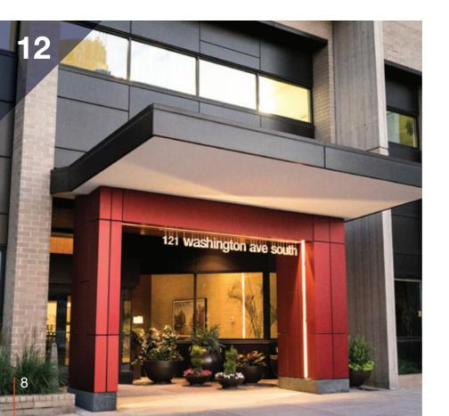
Ranging from a pressure equalized rainscreen system, to a fully caulked barrier wall system or decorative perforated coverings standard construction is with 0.125 plate, ideal for cladding applications that go down to grade or as an accent around an entrance. The panel thickness prevents denting common in thinner rainscreens or ACM panels and eliminates the possibility of delamination.
