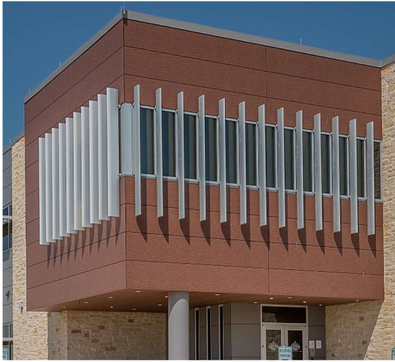
Figure 1.1 - IMP Custom Fit installed
