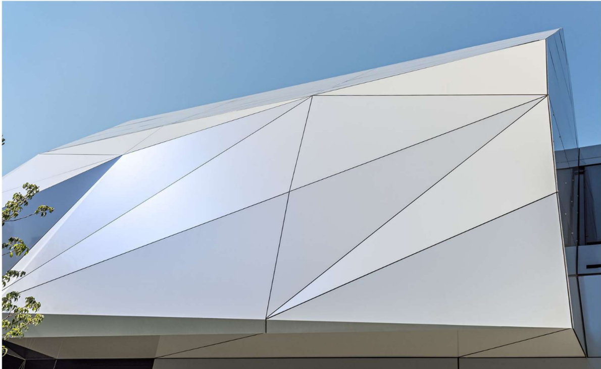
Figure 2.0 – ACM installed
