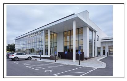
The ACM-3000RS Series is an extruded perimeter **spline joint, back-ventilated rainscreen** panel system, which provides a contemporary look with <u>crisp, caulk free edges</u>. ACM panel systems are best used in low rise applications above grade. The ACM-3000RS system is our <u>lowest cost</u> option for the service life of your project based upon low initial material cost and minimal service cost over the life of the product.
